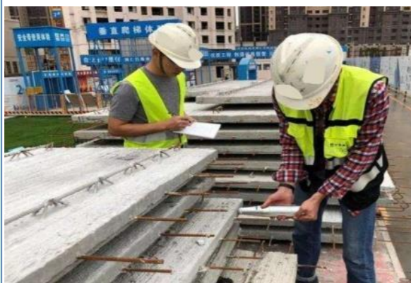
叠合楼板进场验收
