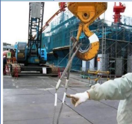
吊具检查合格后方可起吊
