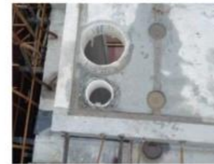
机电结构连接构件优先预留预埋
