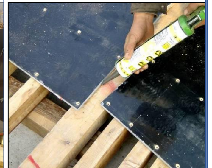
拼缝在龙骨、板缝打胶、钉眼下沉
